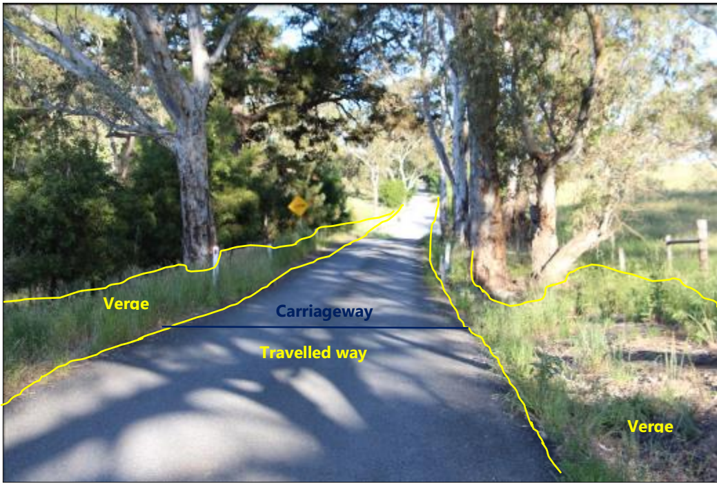
Figure 9: Verge is directly adjacent to the bitumen, and regrowth clearance is restricted to understorey only in this instance. The large trees would not fall under these guidelines and clearance would require an application as they are not considered regrowth under 20 years old.
