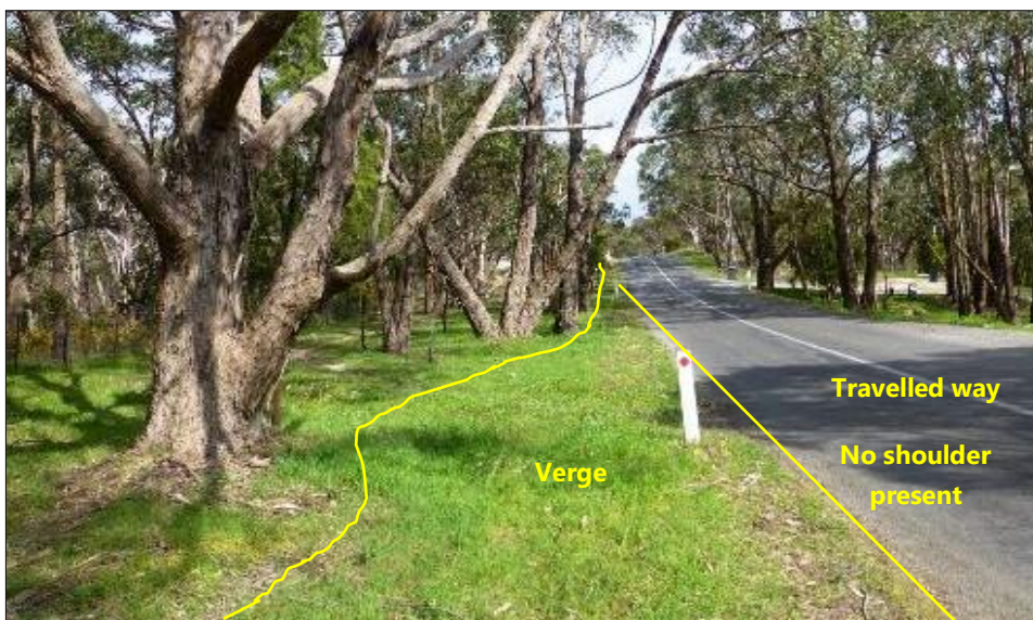
Photo 5. A rural sealed road where a dirt road appears to have been sealed, including the shoulder, therefore the travelled way is directly adjacent the verge.
