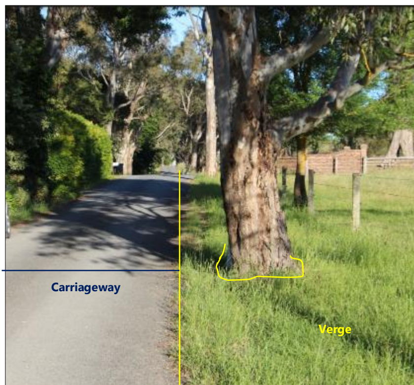
Figure 7: Travelled-way and carriageway are the same width in this instance, with verge regrowth clearance restricted to understorey only.
