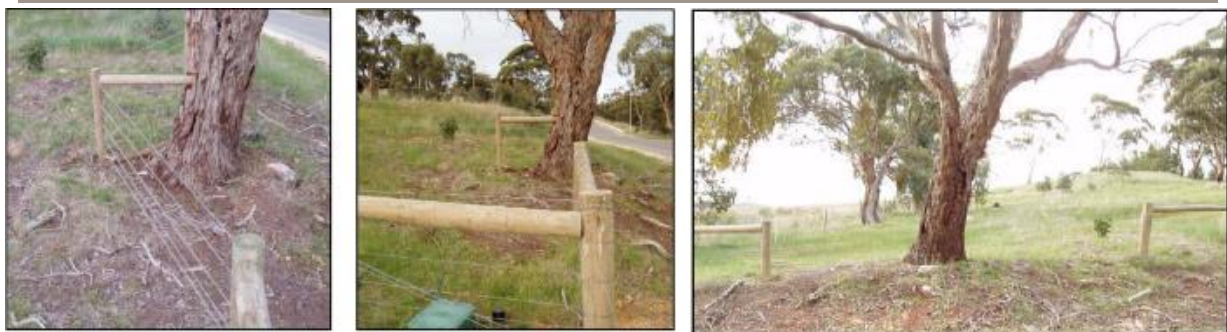
Figure 11. Figure 11. Fenceline strut arrangement. Note: this approach may not be appropriate for smaller trees and an effort should be made to avoid structural roots when placing the post hole for the strut next to the tree.
